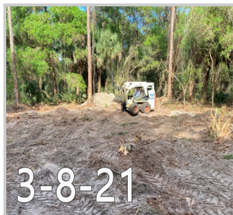
March 2021 ~ Clearing the land took almost two months to clear enough land and bring in fill-dirt to start the foundations of the house and workshop
