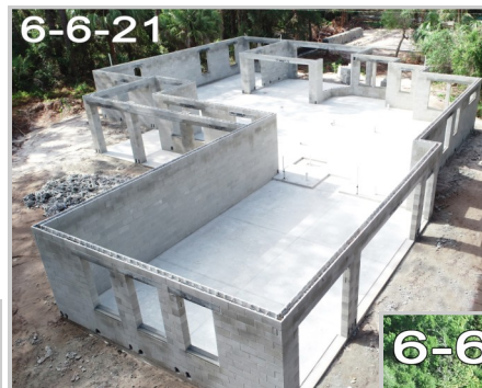
6-6-21: The block walls finally go up for the house
